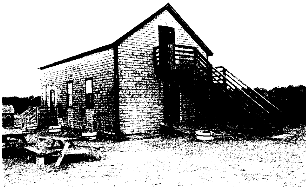
Photo #15 of 17 Stable - south & east elevations
