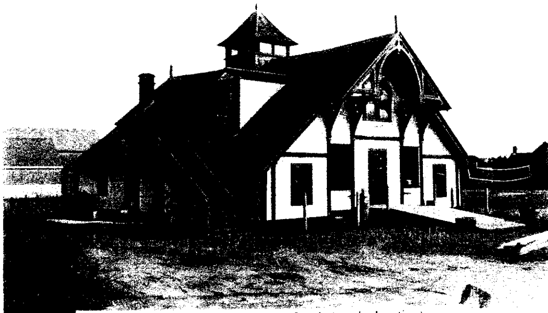
Photo #7 of 17 - west elevation & façade (south elevation)
