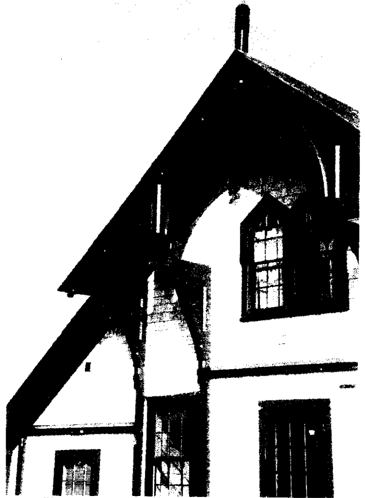
Photo #3 of 17 façade detail of decorative truss
