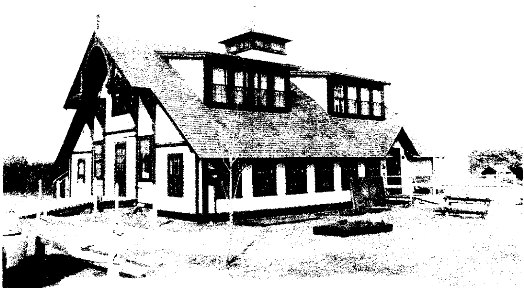
Photo #4 of 17 façade (south) & east elevations of station
