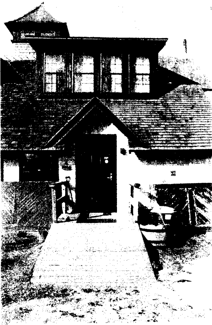
Photo #5 of 17 east elevation entry ramp & dormer
