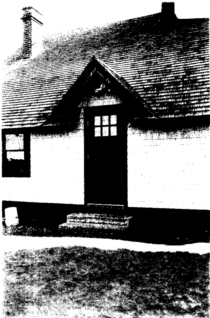
Photo #8 of 17 - west elevation - view of rear entry
