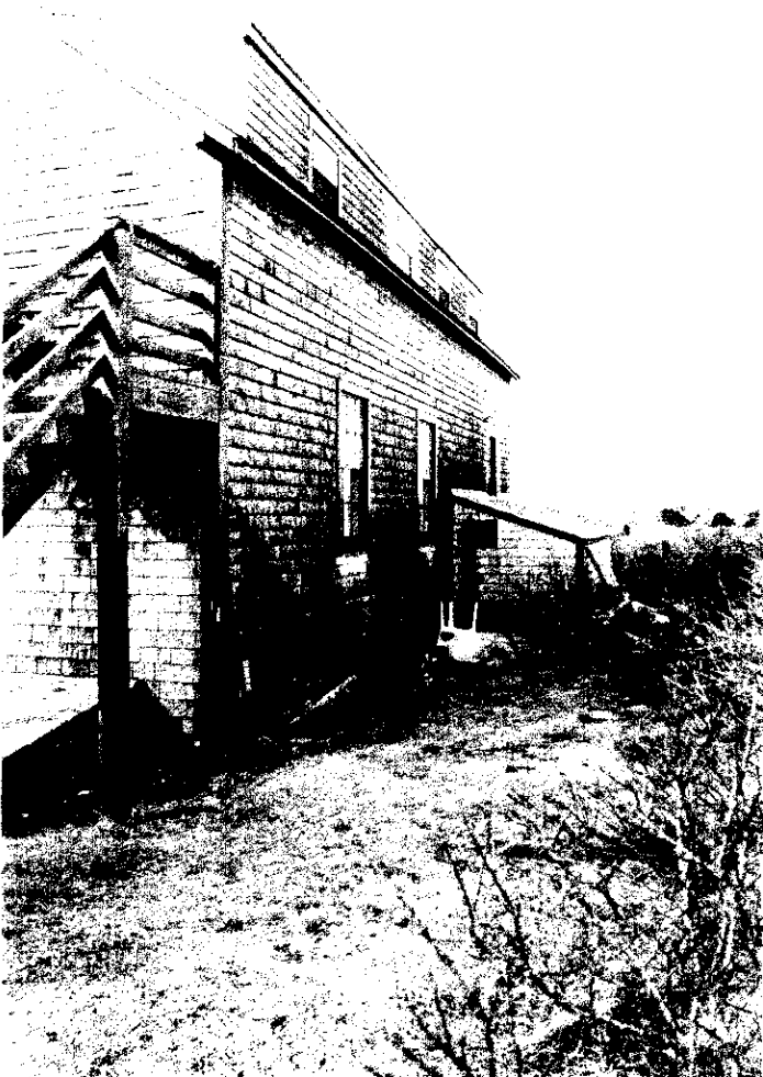
Photo #16 of 17 Stable east & north elevations (left to right)
